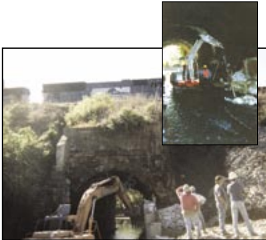
Train bridge underpinning
