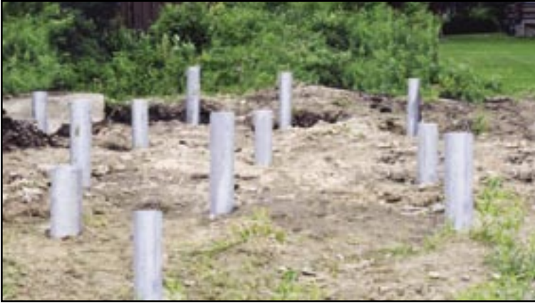
Allows for post-installation depth and plumbness inspection
