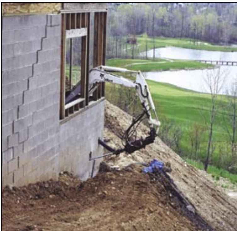
Tie-back anchor installation with difficult access
