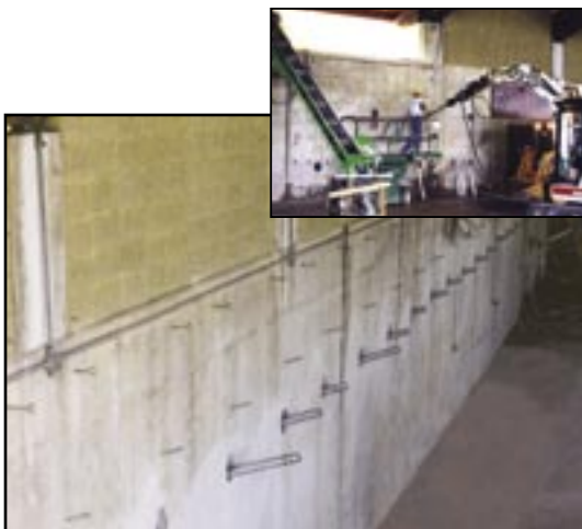
Installation 80 kip tie-back anchors wall stabilization
