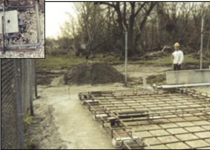
Gridwork for towers
