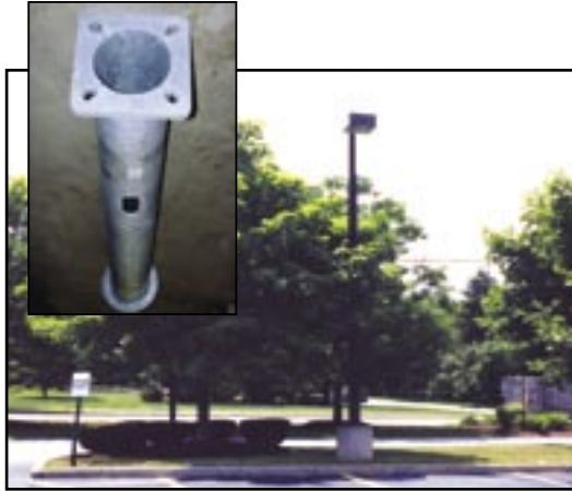
Light pole base
