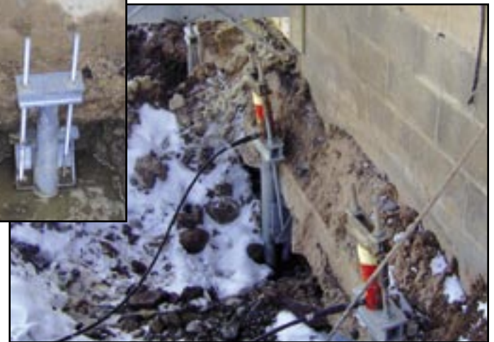
Underpinning commercial building
