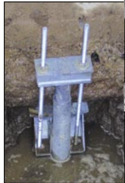
CounterForce™ Underpinning Bracket (patent pending)
