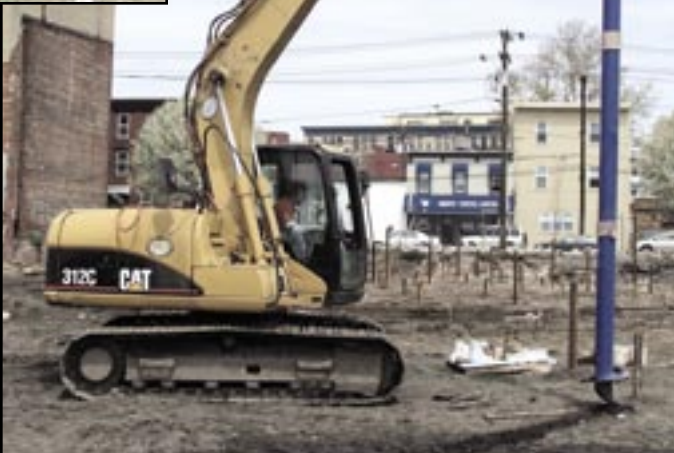
New foundations 40-100 ton capacity
