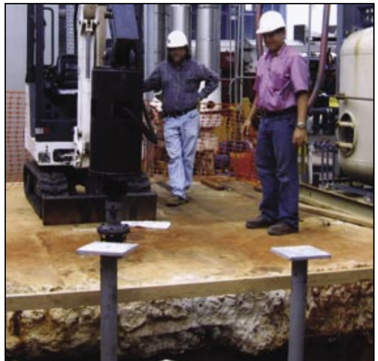
Difficult-to-access and low clearance pharmaceutical structures
